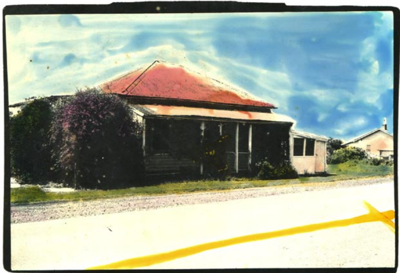
The cottage beside Lawrence Hargrave Drive in upper Coalcliff. Hand-coloured photo - John Dory, 1980
